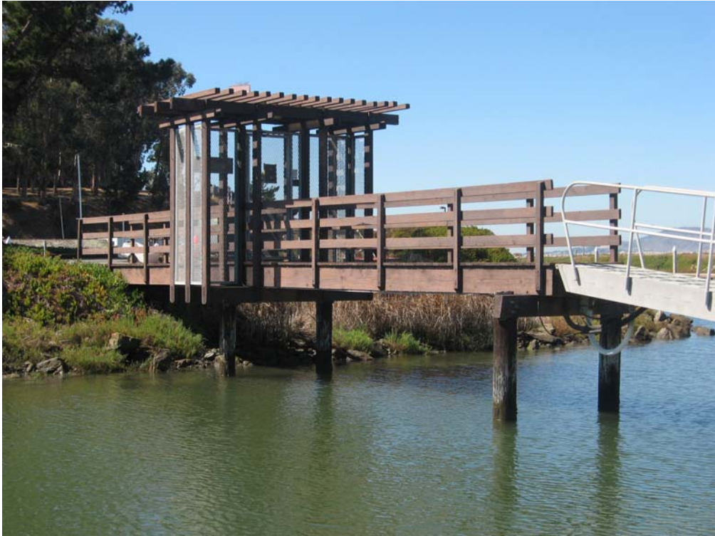
Typical timber piles at gatehouse – wrap timber piles for long term protection
