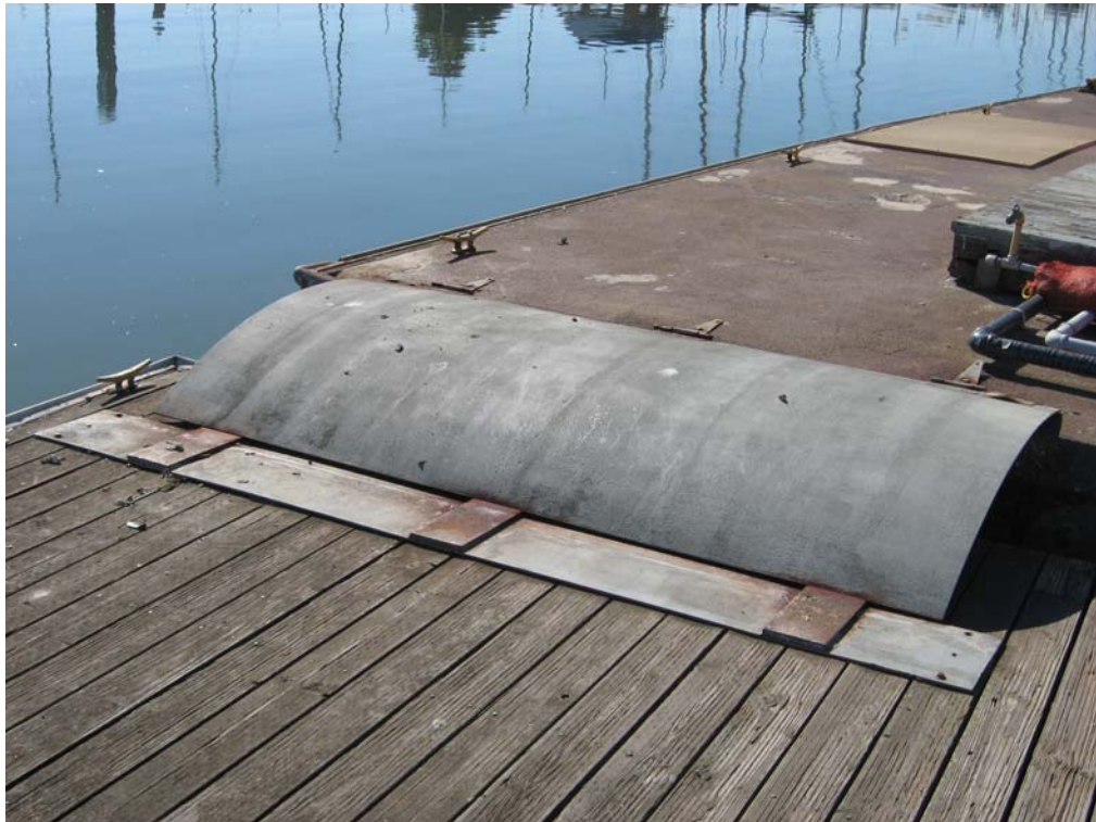
Fuel Dock – Non-standard transition plates.
